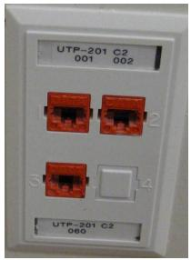
Outlet label placement 4-port: under top-aligned, Plexiglas cover – servicing IDF identifier over port identifiers. Ports should be identified left-to-right. Under bottom-aligned, Plexiglas cover – servicing IDF identifier over port identifiers. Ports should be identified left-to-right. Follow 3-port example.
